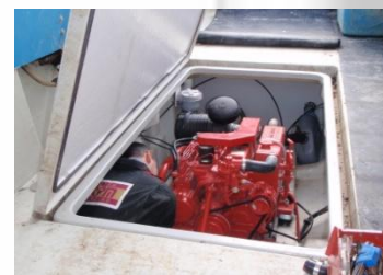
KPM Engineers fit KPM Pumps and strainers
